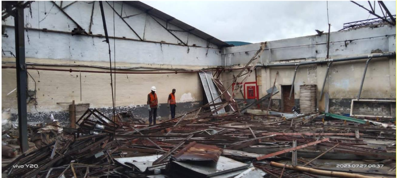
Figure 18: Onsite Demolition of Legacy Industrial Structure at PTHM Unit-2
