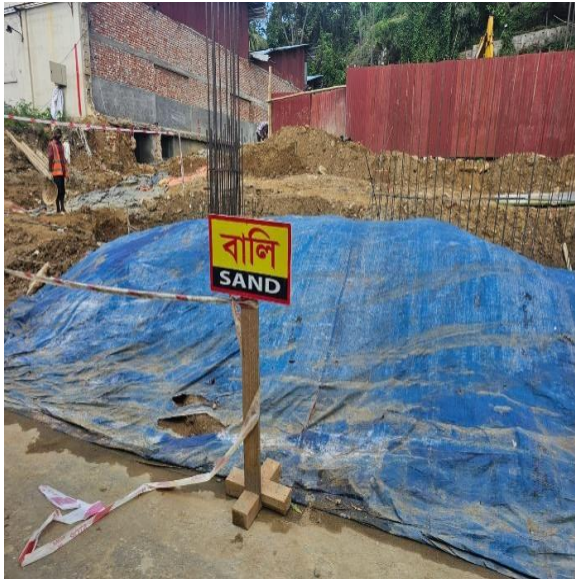
Figure 21: Control of wind erosion and dust generation
