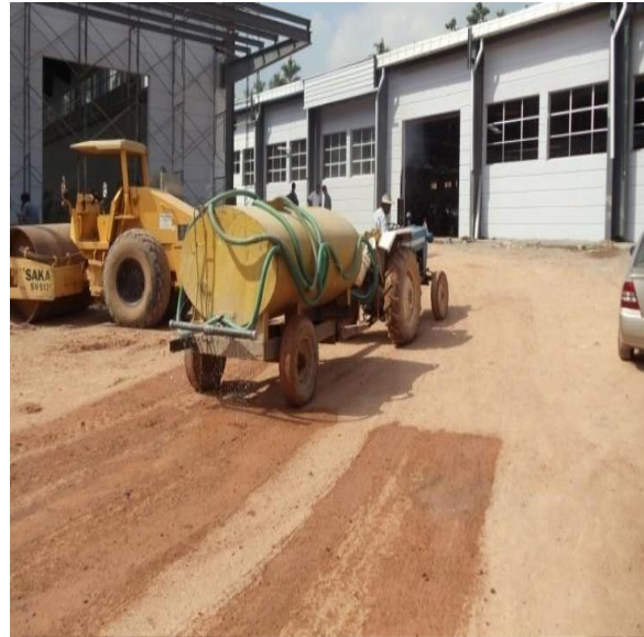
Figure 21: Control of wind erosion and dust generation
