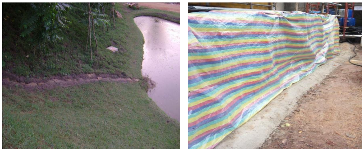
Figure 25: Temporary drains and hums
