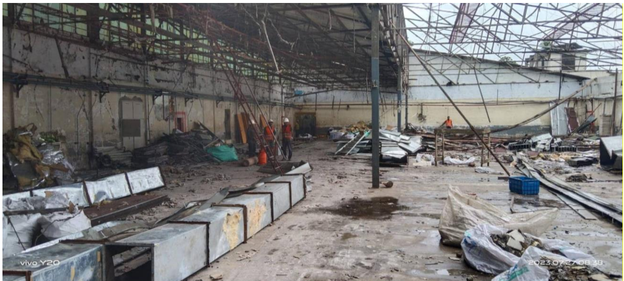
Figure 19: Ongoing Demolition and Material Segregation Activities at Legacy PTHM Unit-2 Building
