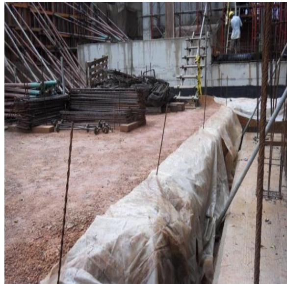
Figure 22: Covered excavated areas and vertical edges
