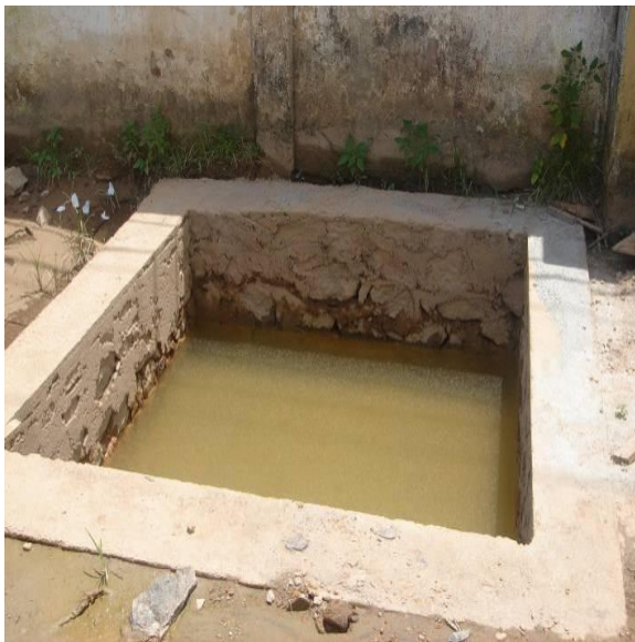
Figure 20: Temporary Sedimentation Chambers
