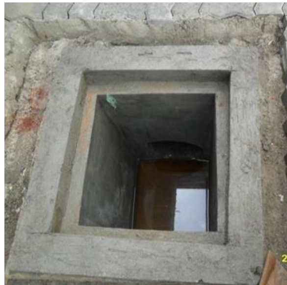
Figure 20: Temporary Sedimentation Chambers
