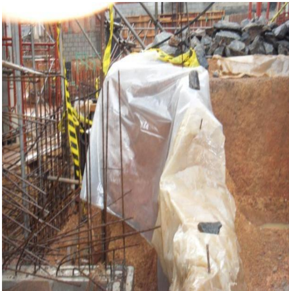
Figure 22: Covered excavated areas and vertical edges
