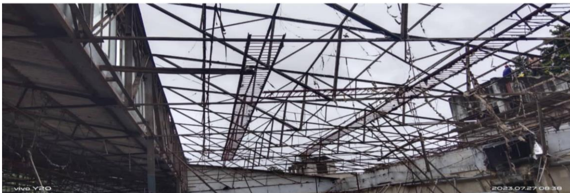
Figure 17: Exposed Steel Truss Framework During Legacy Roof Demolition at PTHM Unit-2
