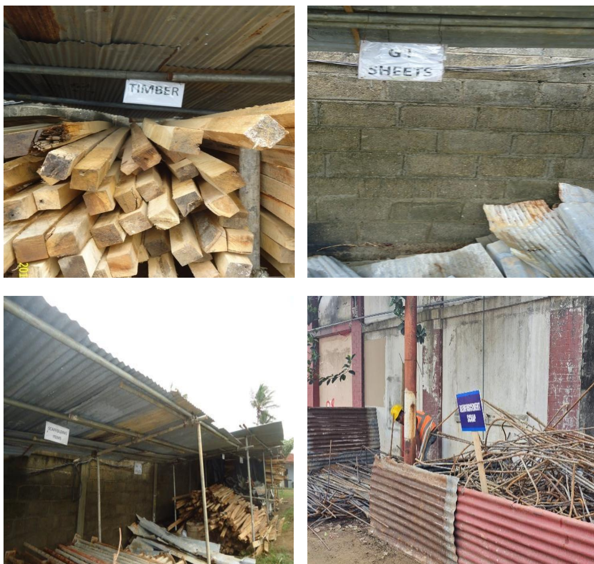
Figure 24: Segregation of waste (Using signing boards)
